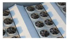
Figure 1. Induced draft air coolers
