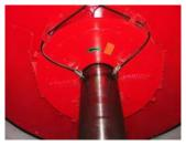
Figure 4. Examples showing sensor installation on the hydro generating units. On the far left is the velocity sensor on the generator top cover for monitoring axial vibrations. The two photos in the middle show the X-Y radial displacement sensors mounted just over the turbine guide bearing. On the far right are the X-Y radial displacement sensors mounted below the lower generator guide bearing.
